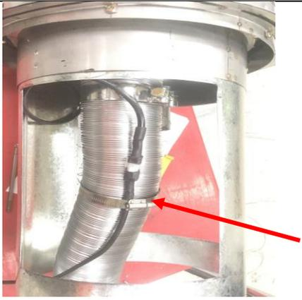
Connect the fan power cable from the appliance to the termination.
