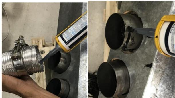
On the heater connection end - Fit clamp loosely & apply silicon inside the pipes. Apply an 8mm silicon bead fully around the inside of the flue and on the heater spigot. Smear the silicon around the spigot and pipe.
